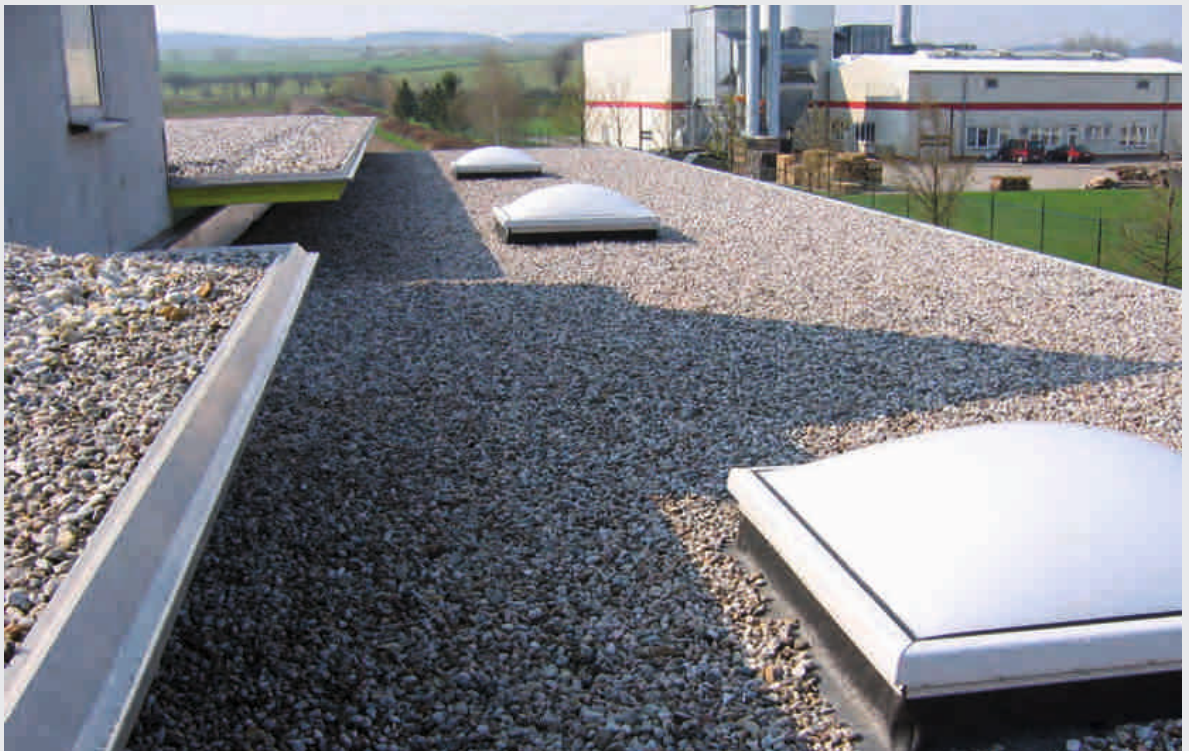
Flat roof with a gravel protection layer
